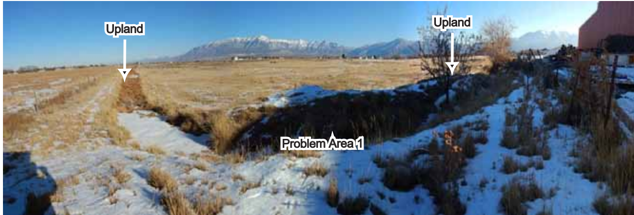
Photo 17. Northeast view of excavated, man-made irrigation Ditch 1 in the southwest corner of the Project Area. It appears Ditch 1 flows in a north/south direction along the west Project Area boundary before turning eastward along the south Project Area boundary. The ditch has been excavated several feet lower than the native ground elevation.
